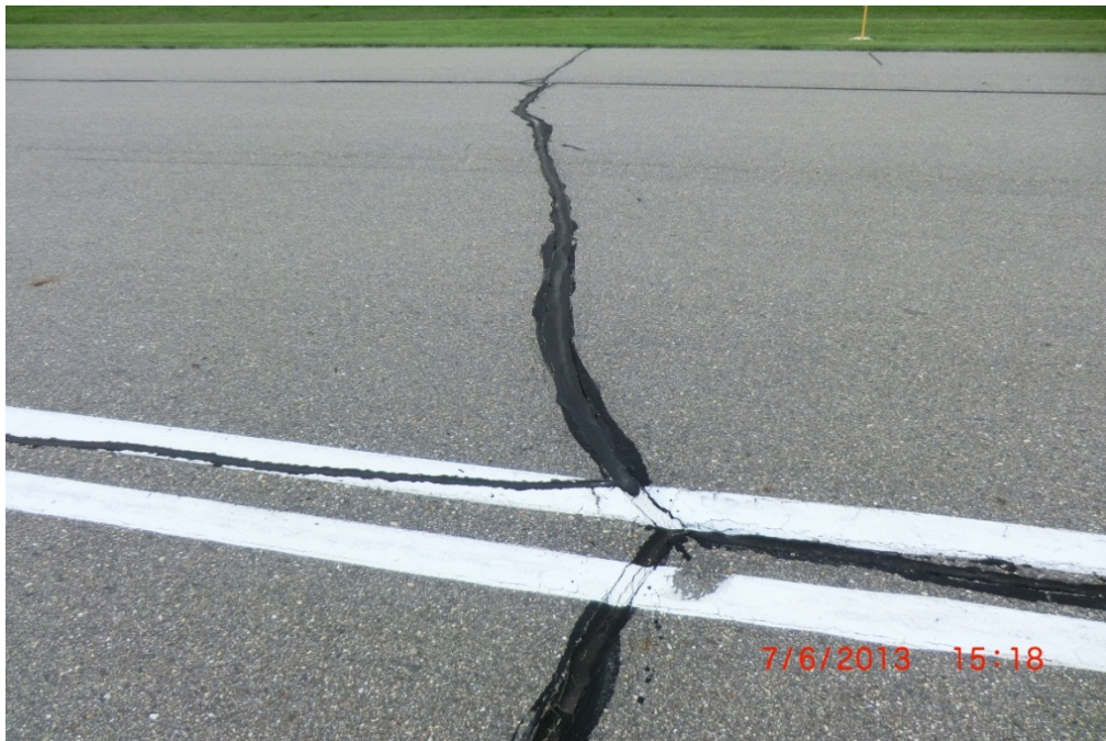
7Y4 RY1432 001 (High Severity L&T Crack)
