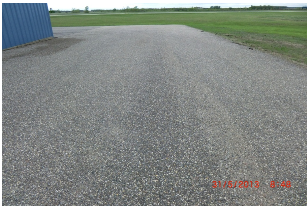
16D TLA 002 (PCI = 23, Several Distress Types Not Visible in Photo)
