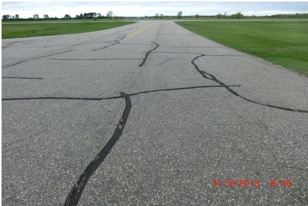
16D CTA 002 (PCI = 36, Several Distress Types Not Visible in Photo)
