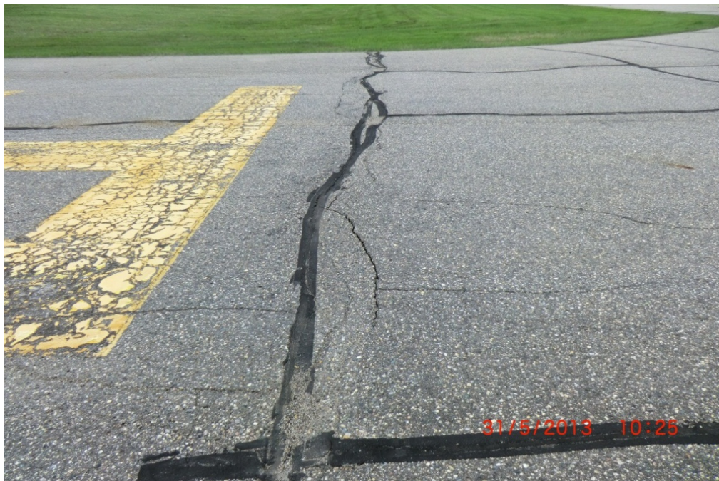
16D APA 001 (High-Severity L&T Crack)
