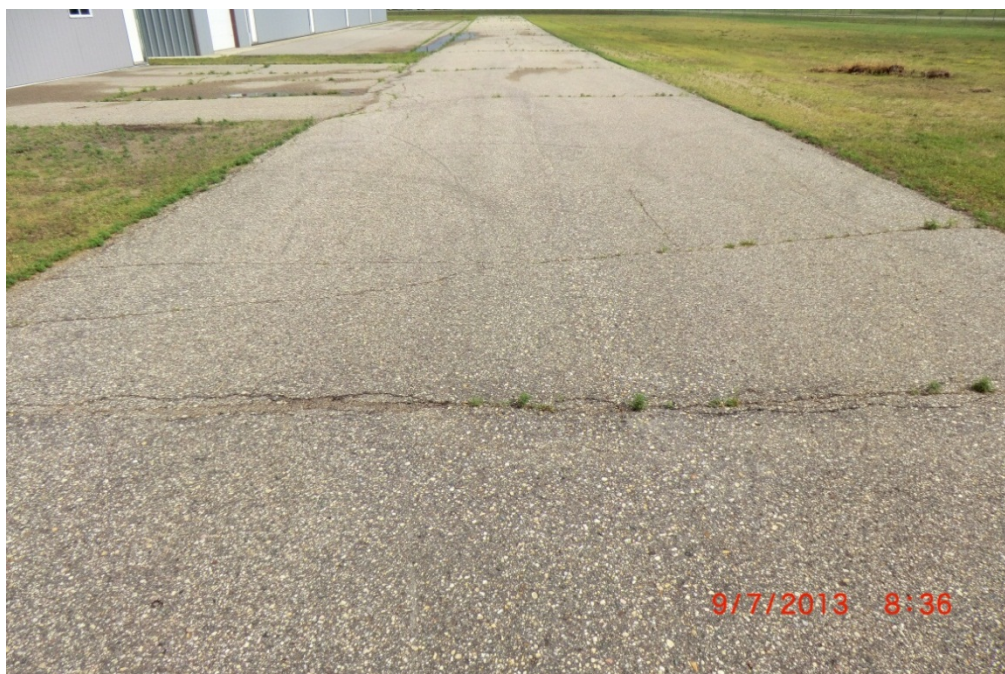
14Y TLA 002 (PCI = 36, prior to rehabilitation)
