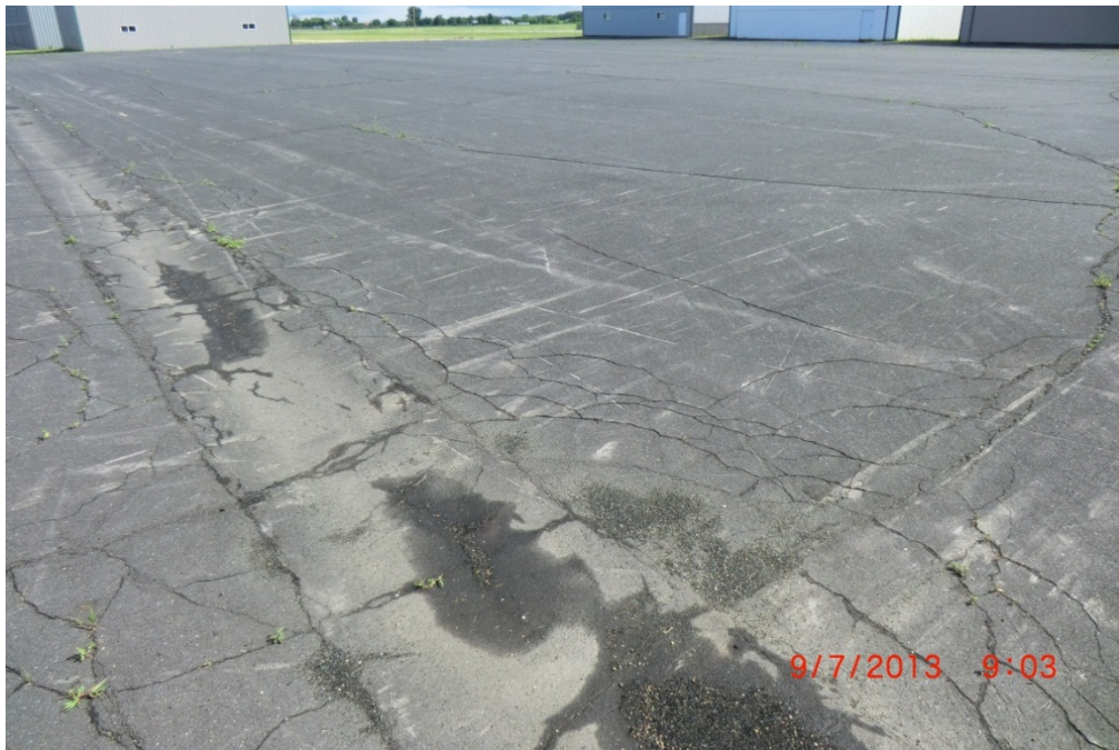
14Y APA 002 (PCI = 57, prior to rehabilitation)
