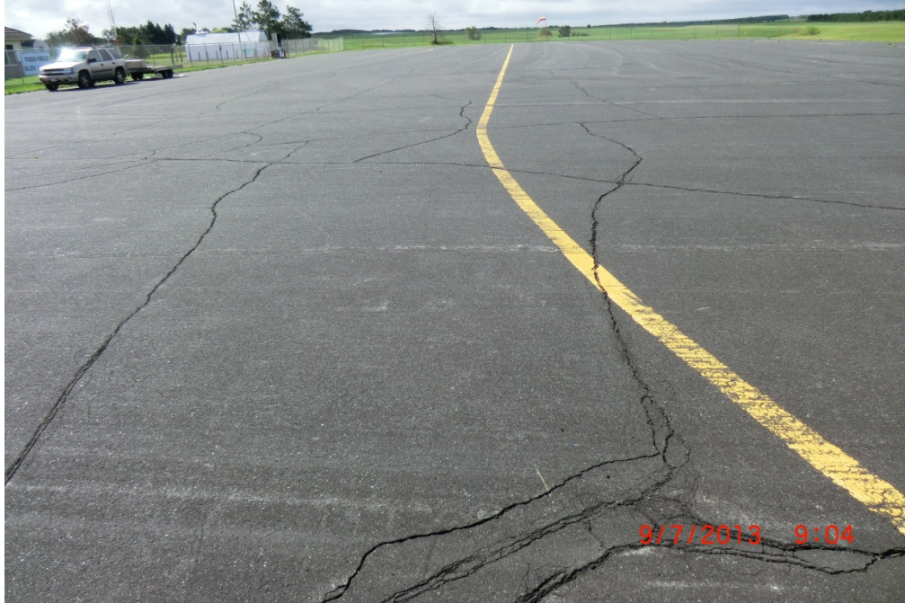
14Y APA 001 (PCI = 58, prior to rehabilitation)
