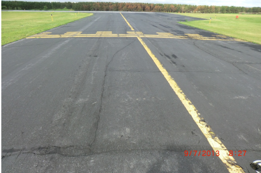
14Y CTA 001 (PCI = 57, prior to rehabilitation)
