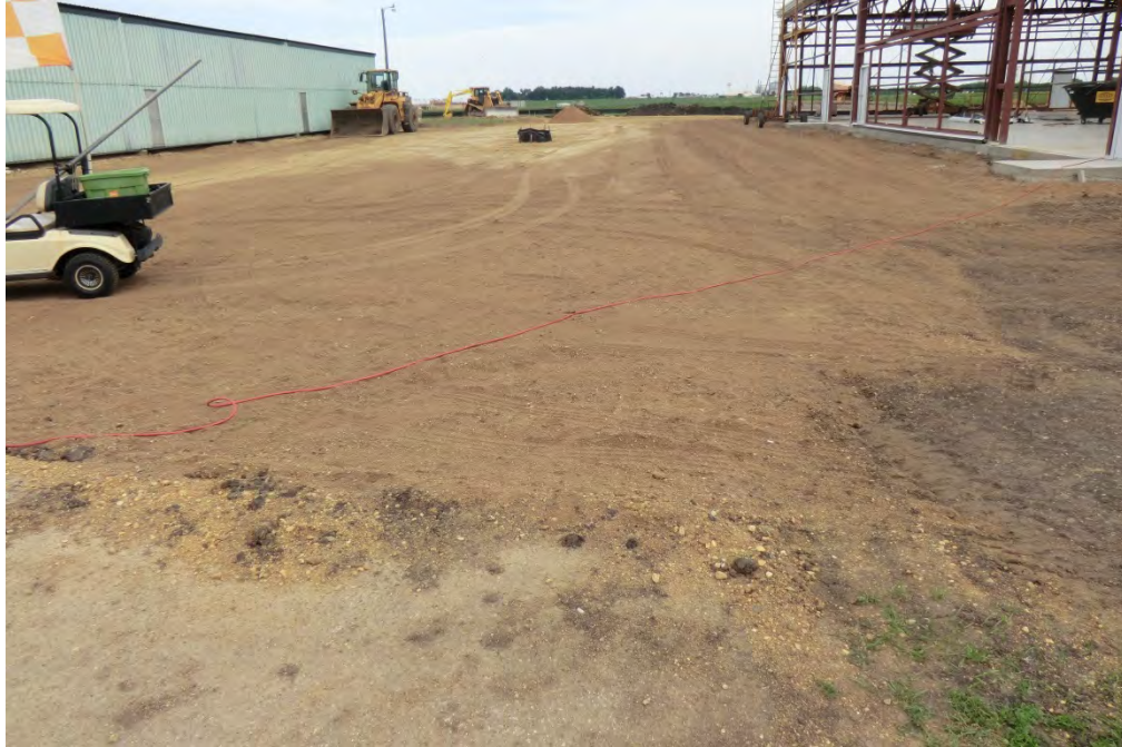
OTG TLA 004 during construction
