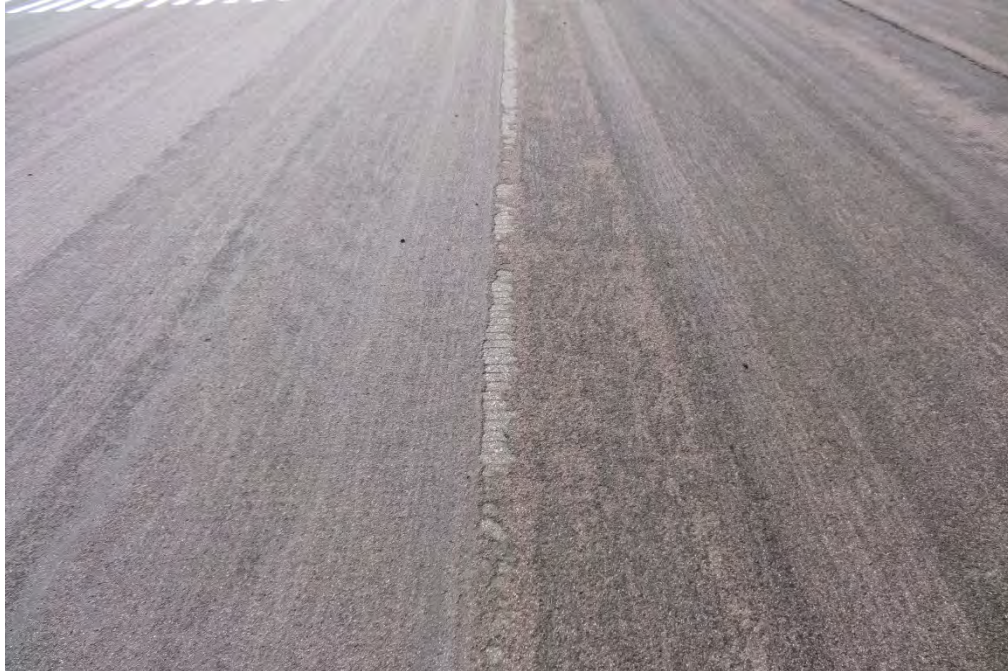
OTG RY1129 001 slurry seal, (PCI = 80)
