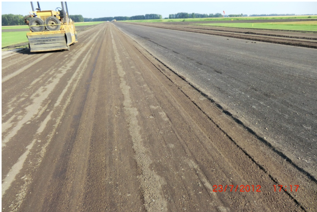
D37 RY1230 001 during construction
