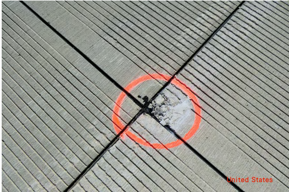
STC RY1331 001 Corner spall, (PCI = 98)
