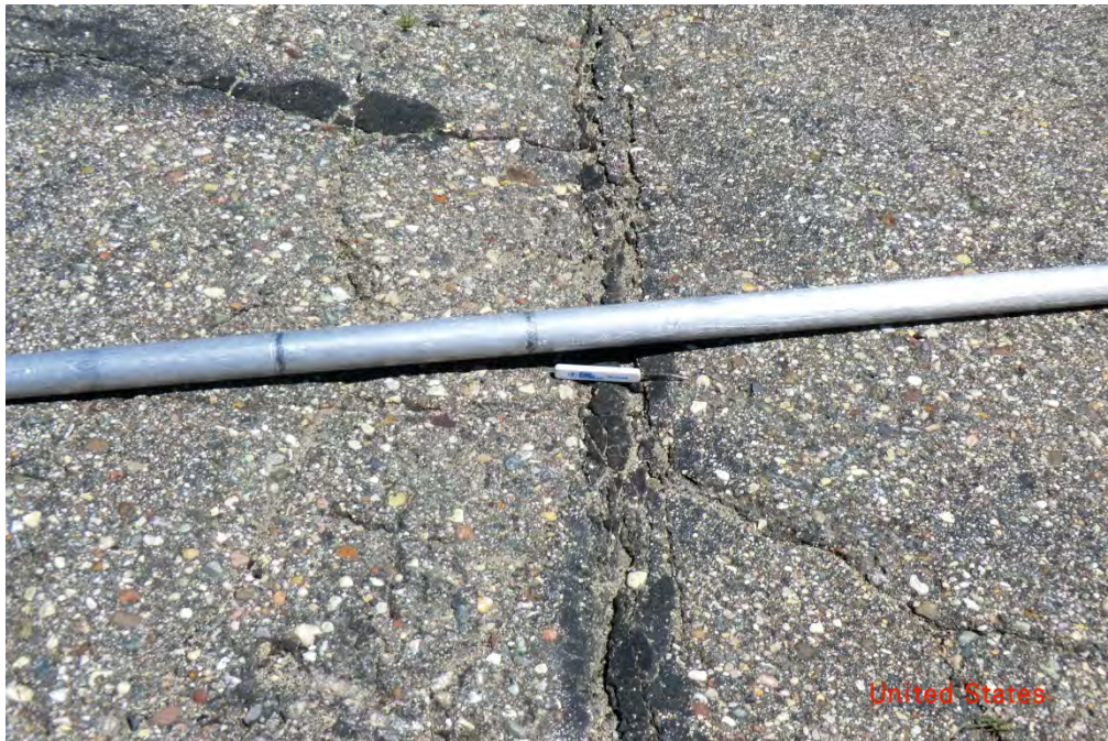
STC TLA 001 Rutting, (PCI = 20)
