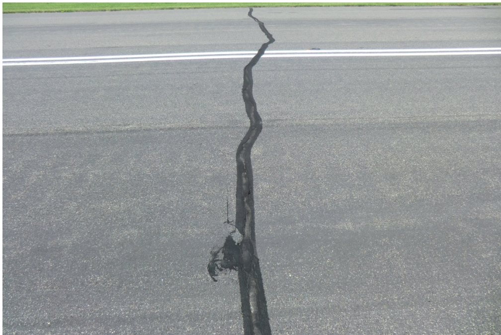
55Y RY1634 001 crack seal (PCI = 89)
