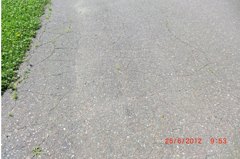
ROS TLA 001 Alligator Cracking, (PCI = 25)
