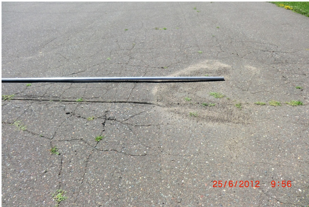
ROS TLA 001 Alligator Cracking & Rutting, (PCI = 25)
