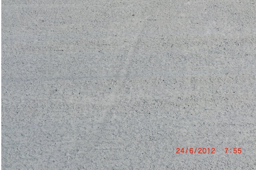
PEX RY1129 001 L & T Crack under slurry seal, (PCI = 95)
