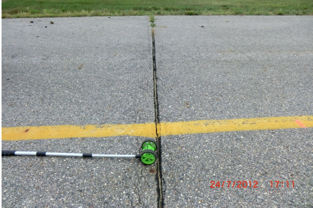
JKJ CTA4 001 L & T Cracking, (PCI = 84)
