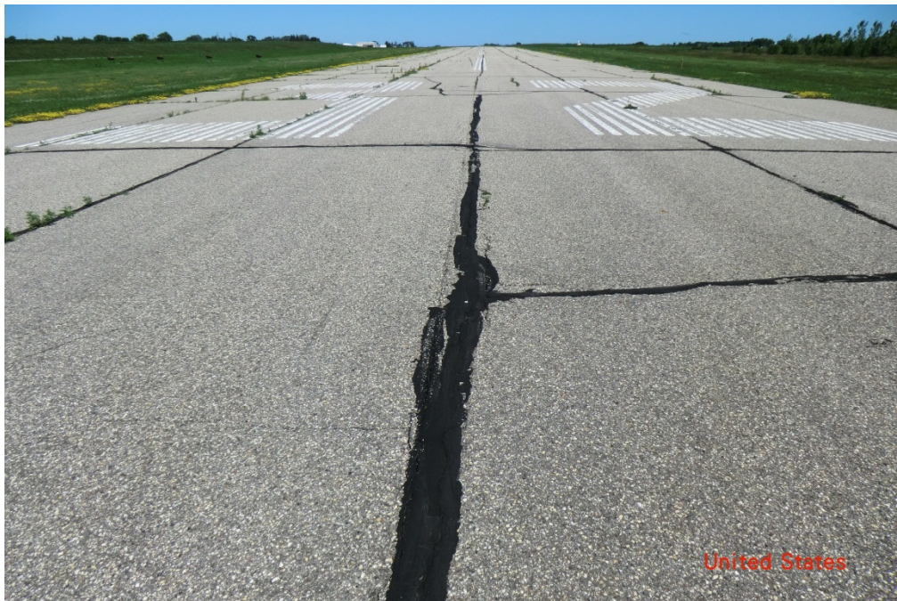
MVE RY1432 002 (prior to rehabilitation)
