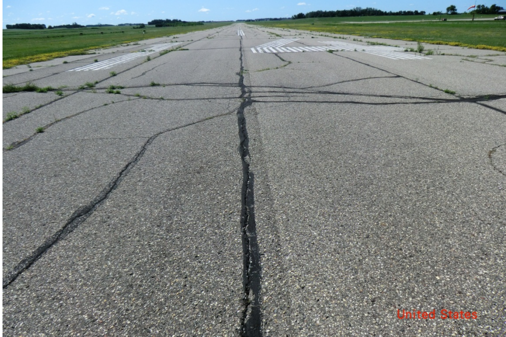
MVE RY1432 001 (prior to rehabilitation)
