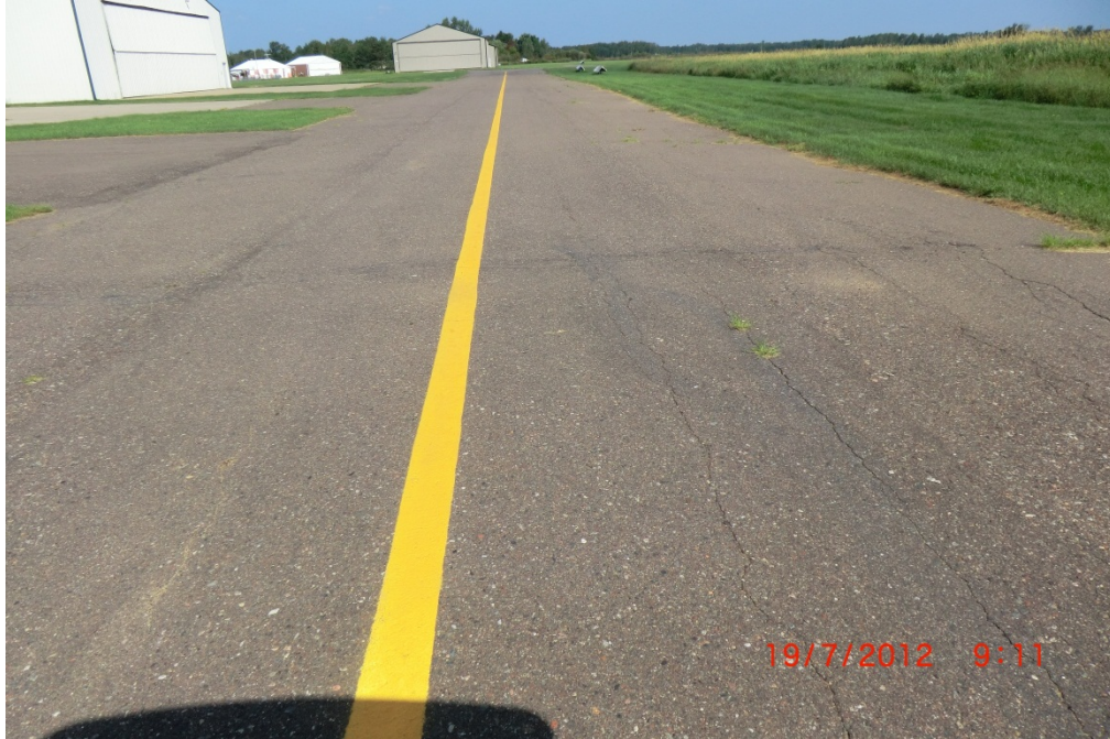
HZX TLA 001 (prior to rehabilitation)
