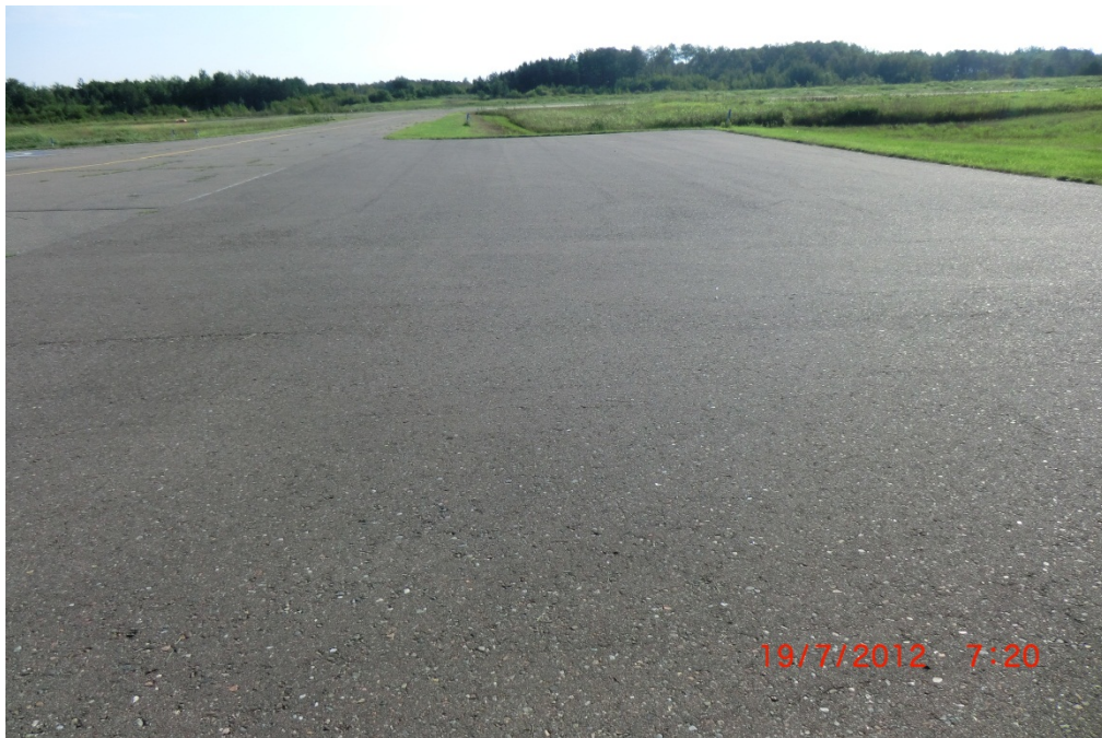
HZX APA 002 (prior to rehabilitation)
