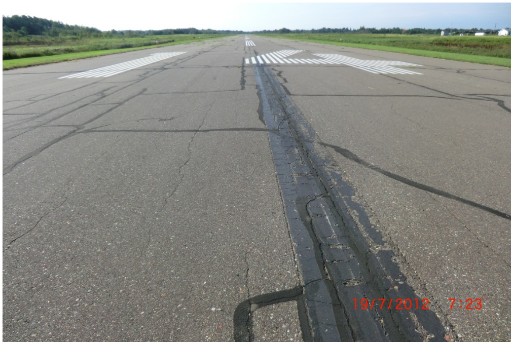
HZX RY1432 001 (prior to rehabilitation)
