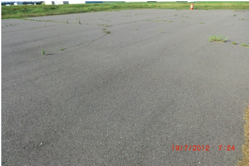
HZX RTA 001 (prior to rehabilitation)
