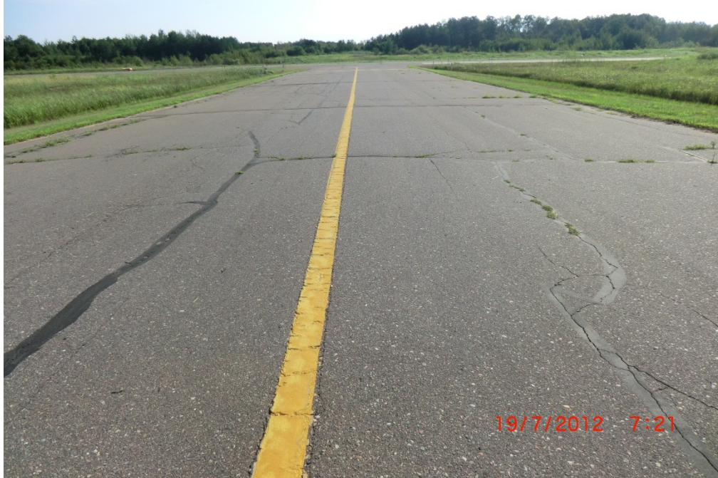
HZX CTA 001 (prior to rehabilitation)
