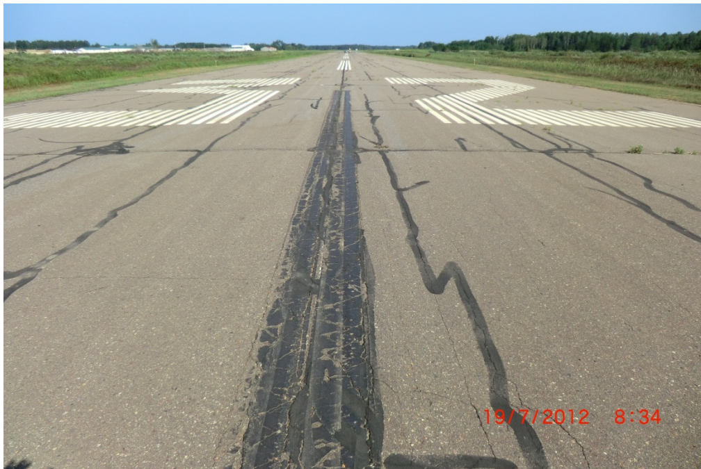
HZX RY1432 001 (prior to rehabilitation)
