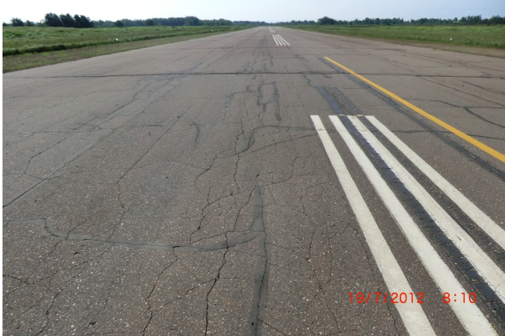
HZX RY1432 001 (prior to rehabilitation)
