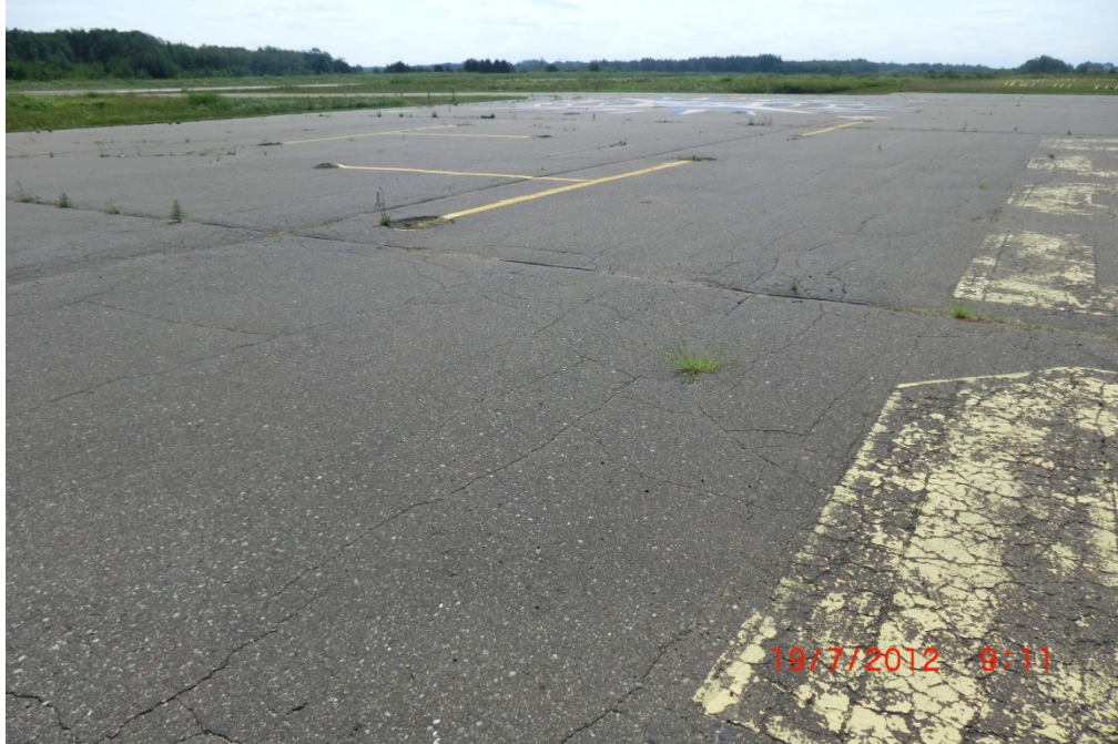
HZX APA 001 (prior to rehabilitation)
