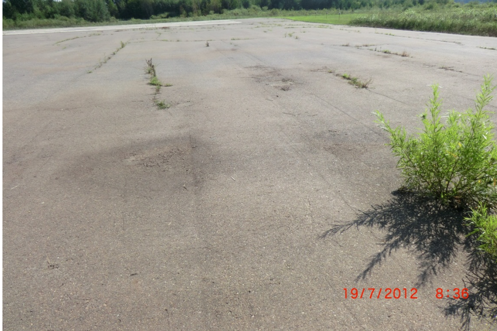
HZX RTA 002 (prior to rehabilitation)
