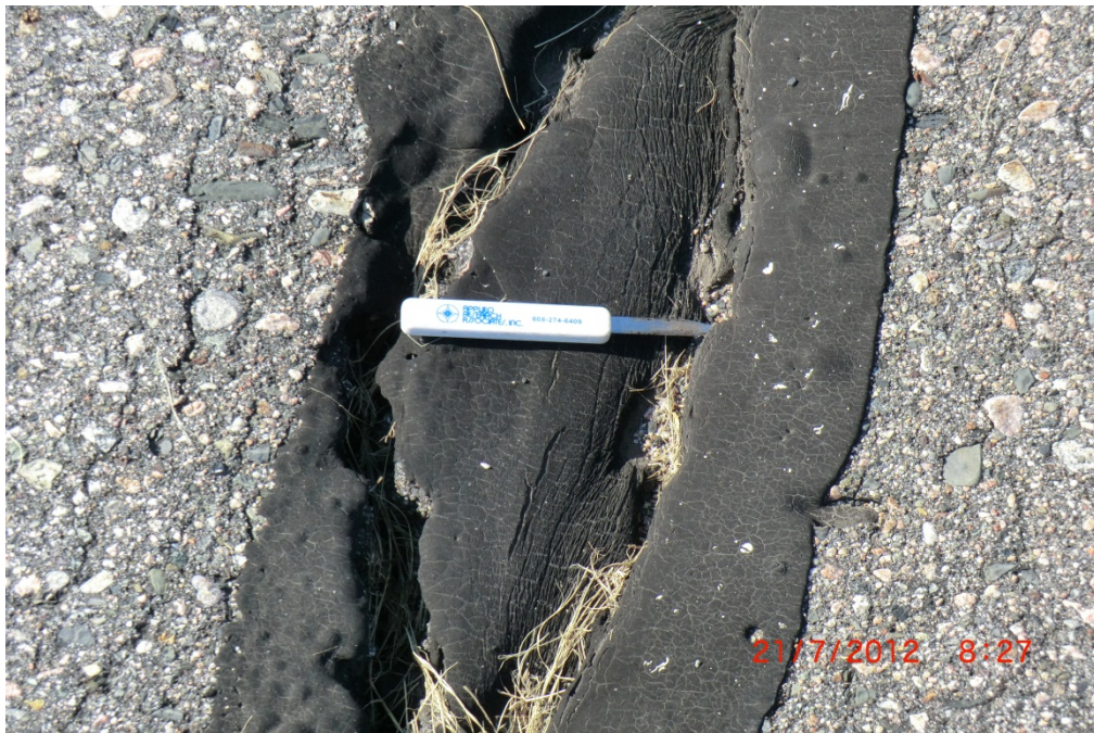
EVM RY927 001 L & T Cracking, (PCI = 43)
