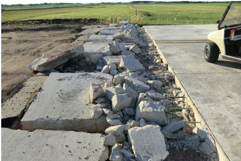
SBU CTA 002 (prior to construction)
