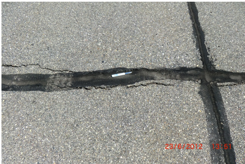
BBB RY1432 003 high severity crack (PCI = 74)
