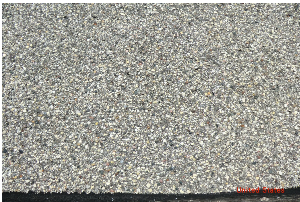
AQP RY1331 001 medium severity raveling (PCI = 27)
