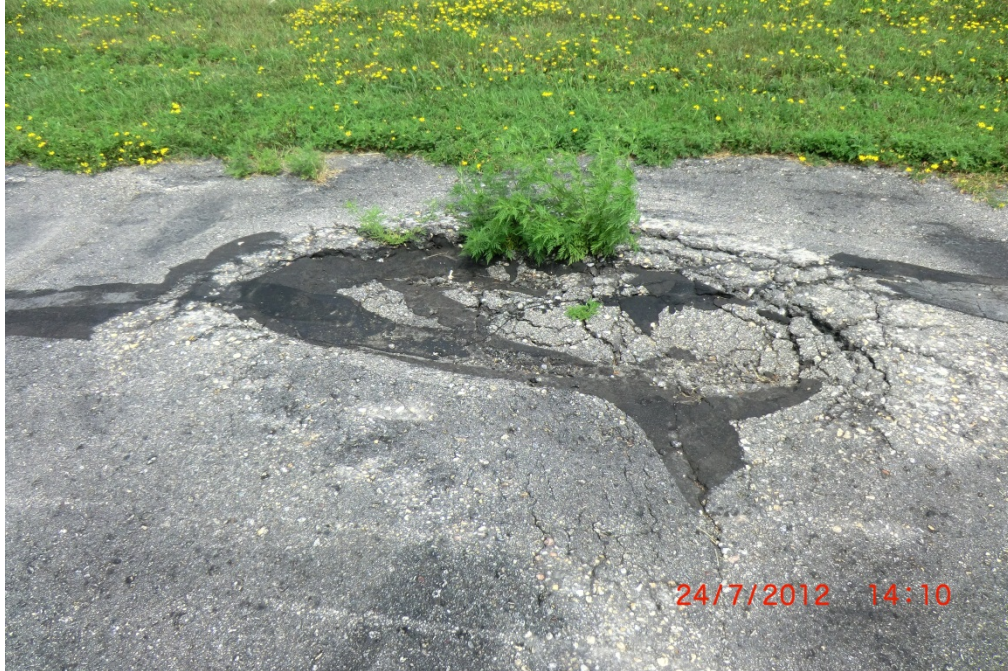
D00 TLA 001 swell & alligator cracking (PCI = 59)
