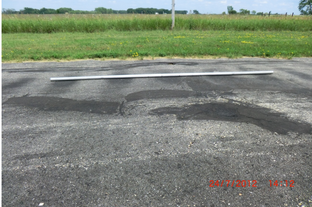
D00 TLA 011 corrugation (PCI = 59)
