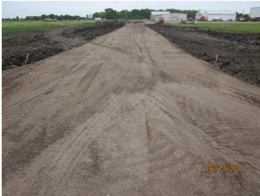
FBL TLF 001 prior to asphalt placement (post construction PCI = 100)
