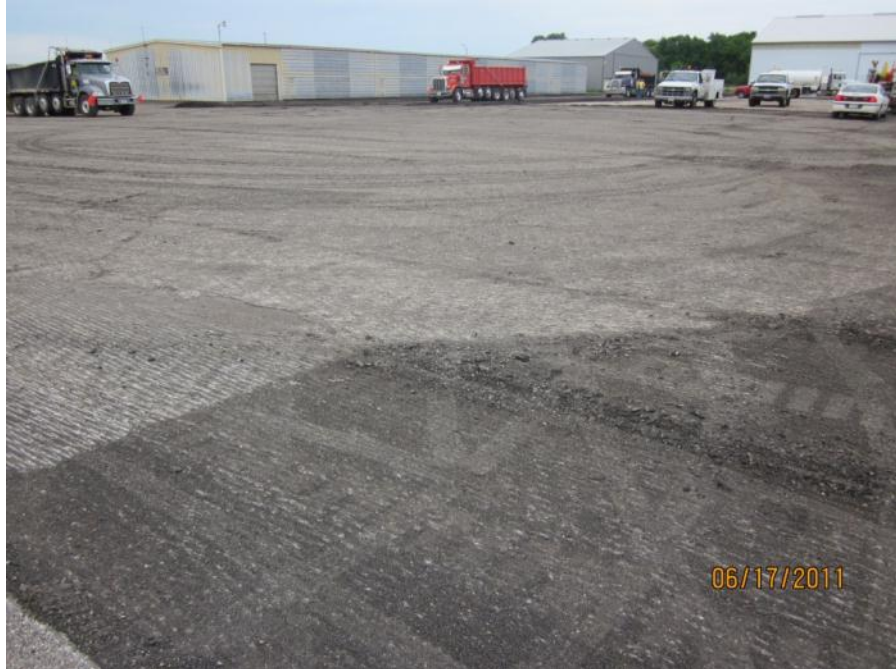
FBL APA 001 – prior to asphalt overlay (post construction PCI = 100)
