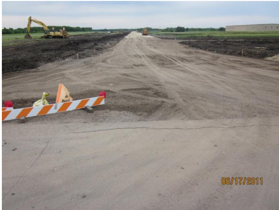
FBL PPTA 001 – prior to asphalt placement (post construction PCI = 100)
