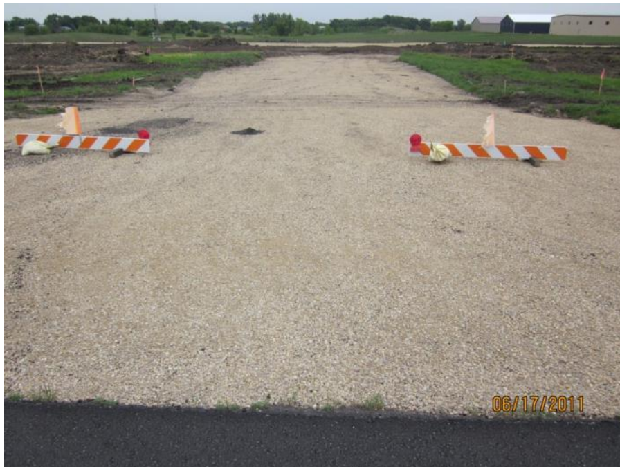
FBL CTC 001- prior to asphalt placement (post construction PCI = 100)
