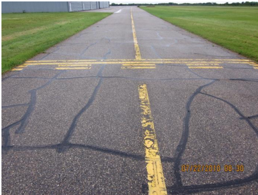
AEL CTB 001 (PCI = 44 prior to 2011 construction)
