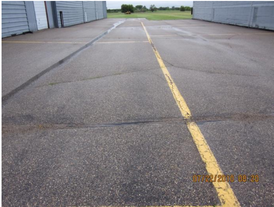
AEL TLB 001 (PCI = 64 prior to 2011 construction)
