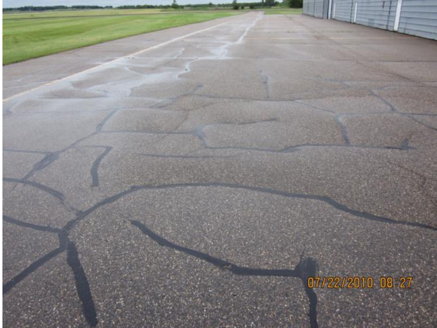
AEL CTB 002 (PCI = 56 prior to 2011 construction)
