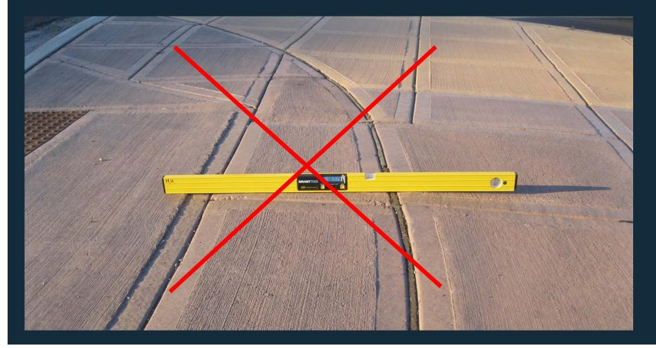
Contraction joints shall extend to at least 30% of sidewalk thickness. If saw cutting provide 1/8 inch wide contraction joint as per MnDOT 2521
