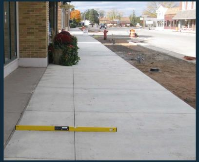
When greater than 50' of continuous sidewalk runs are constructed the contractor shall saw cut all joints.
