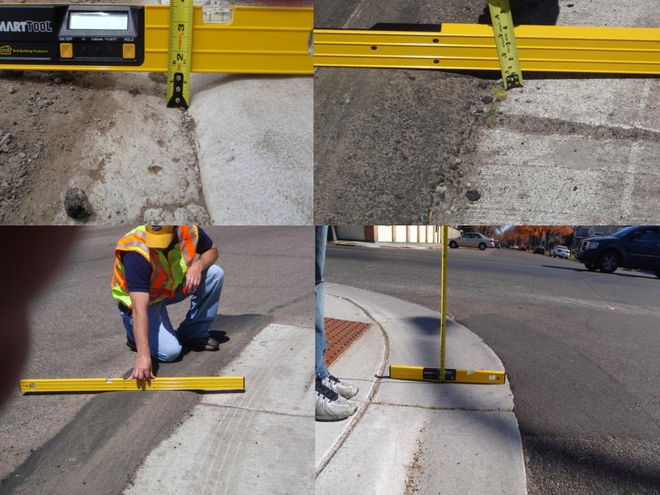
When adjacent to pavement, flares should be constructed at a 10% slope
