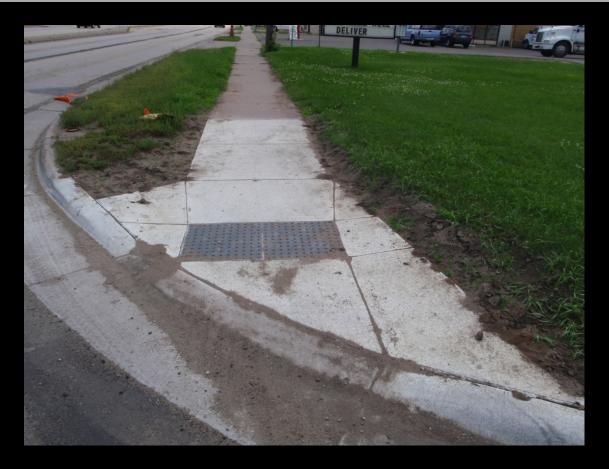
Construct a 2 foot flare to hold back adjacent ground
