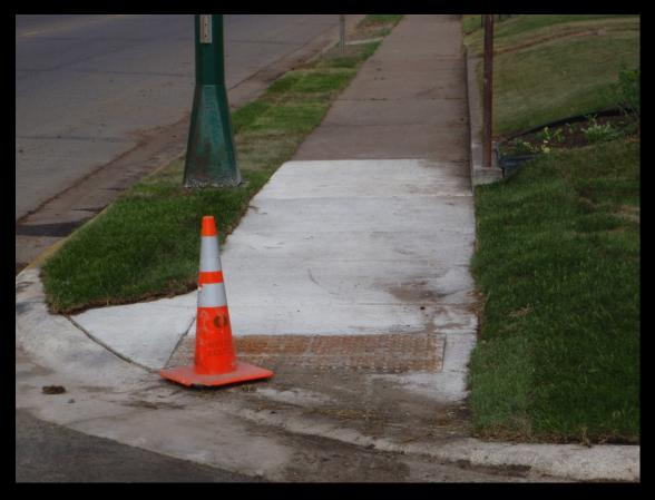
Grade adjacent ground to match new walk and curb and gutter
